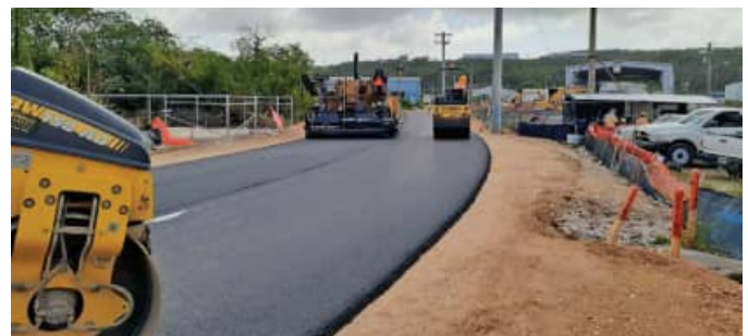
Photos: Harmon Industrial Park Roadway Rehabilitation and Improvement Monthly Reports (No. 1 & No. 2)
